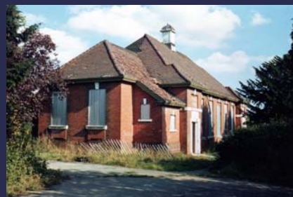
The Assembly Hall, ready for demolition in the late 1980s.
