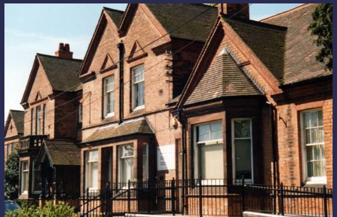
The buildings of Erdington Cottage Homes are still standing, but now have private residents. [MS 2838/4/1/43]
