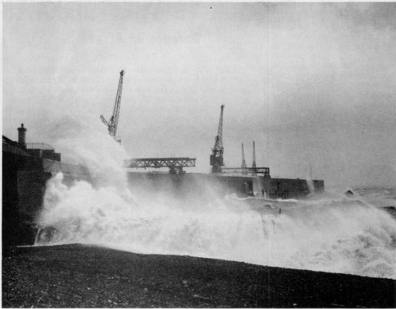
This dramatic photograph, taken at Folkestone harbour, illustrates the kind of conditions which our surface coating treatments must withstand. The cranes in the photograph were treated with Evoled|Evodyne|Evodyne T.C.R. system
