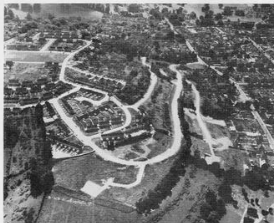
An aerial view of roads in a new housing development at Windmill Hill, Glastonbury, Somerset. Resilex and Evolastik were used for all expansion joints. Contractors—Ruddle Brothers, Civil Engineers and Contractors for the Glastonbury Borough Council. (Evomastics Ltd.)
