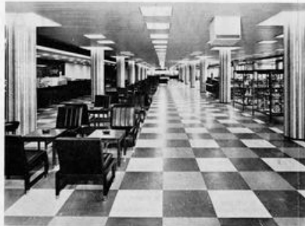
The waiting hall at Oslo Airport. Floor covering PVC tiles by Rickett Floor Tiles manufactured by Reber & Son Ltd. bonded with Evo-stik Floor Adhesive 873. The total floor area covered is approximately 12,000 square metres. Photograph by courtesy of Evonor Ltd., Norway
