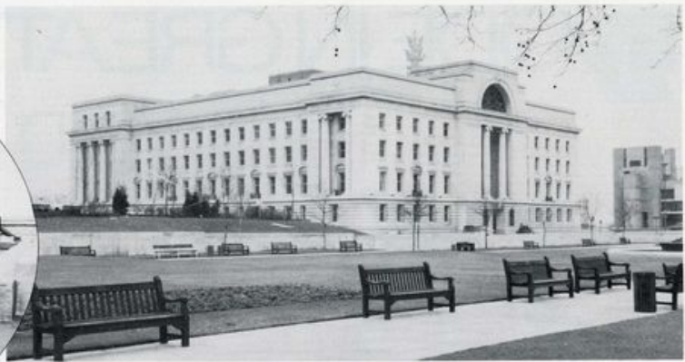
Baskerville House in Birmingham which has been recently waterproofed by Evode Roofing Limited.
