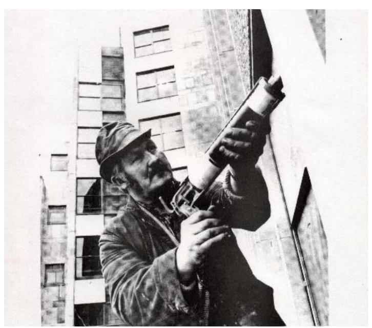
Evode Waterproofing Systems Limited have completed a contract involving the sealing of a 30,000 ft run of  $\frac{1}{2}$  in and  $\frac{3}{8}$  in vertical and horizontal expansion joints incorporated in the new and impressive Douglas House office and shopping complex which has recently been constructed in Newcastle-upon-Tyne city centre.
