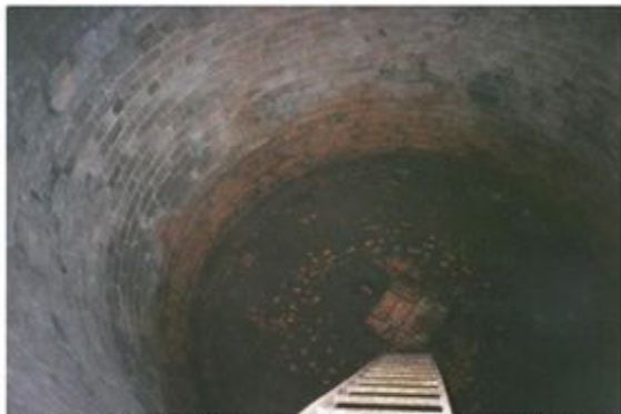
Looking down on the floor of The Ice House. There was a drain in the centre of the floor – it can be seen in the picture near the foot of the ladder. Photo John Walker 1992.
