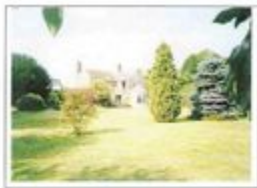
The south-east facade
