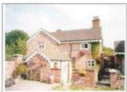
Rear elevation and courtyard
