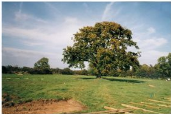
The raised footpath over the Lord's Meadow to the site of Crakemarsh Church. Part of the new road to Rocester is under construction in the foreground (1988). The new road was built to the south of Crakemarsh and bypassed Combridge. The huge beech tree died a couple of years later due – I think – to drought. Photo John Walker 1988.
