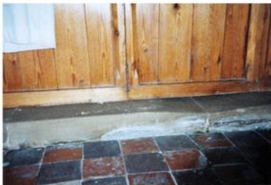
The worn steps in Stramshall church. The well-worn reverse side and its infilling can clearly be seen. Photo John Walker 1990.
