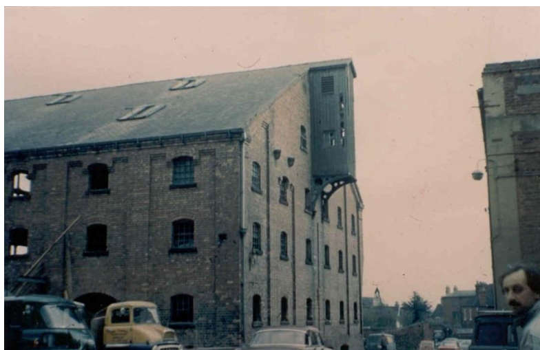
The old Bunting's Brewery just before it was demolished.
